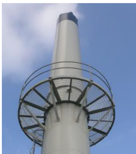
Access platform for emissions monitoring testing – Thermo Technology Ltd
