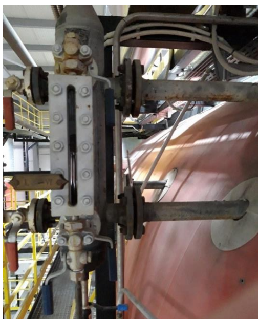
Sight glass installation - Emerson Process Management
