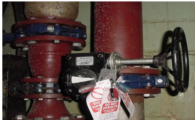
Isolation point locked and labelled
