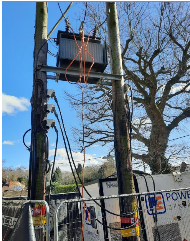
Rural distribution transformer with HV temporary earths and LV generator
