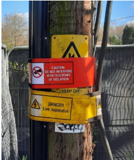
HV Isolation labelling
