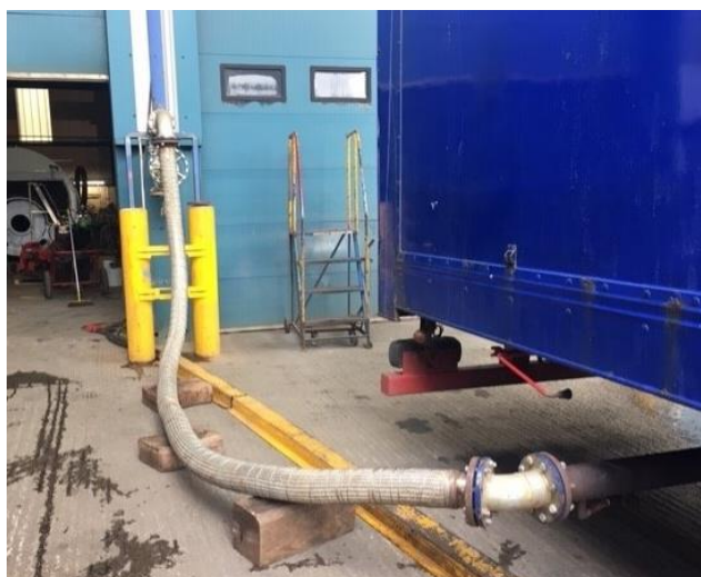
Typical steam hose installation
