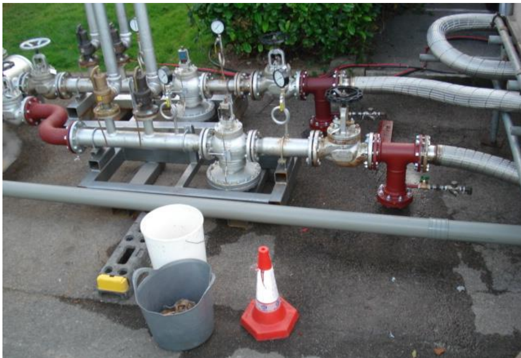
Pressure reducing set under construction.
