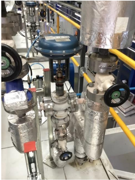
Left 3-way valve installation (Thermal Fluid Solutions)
