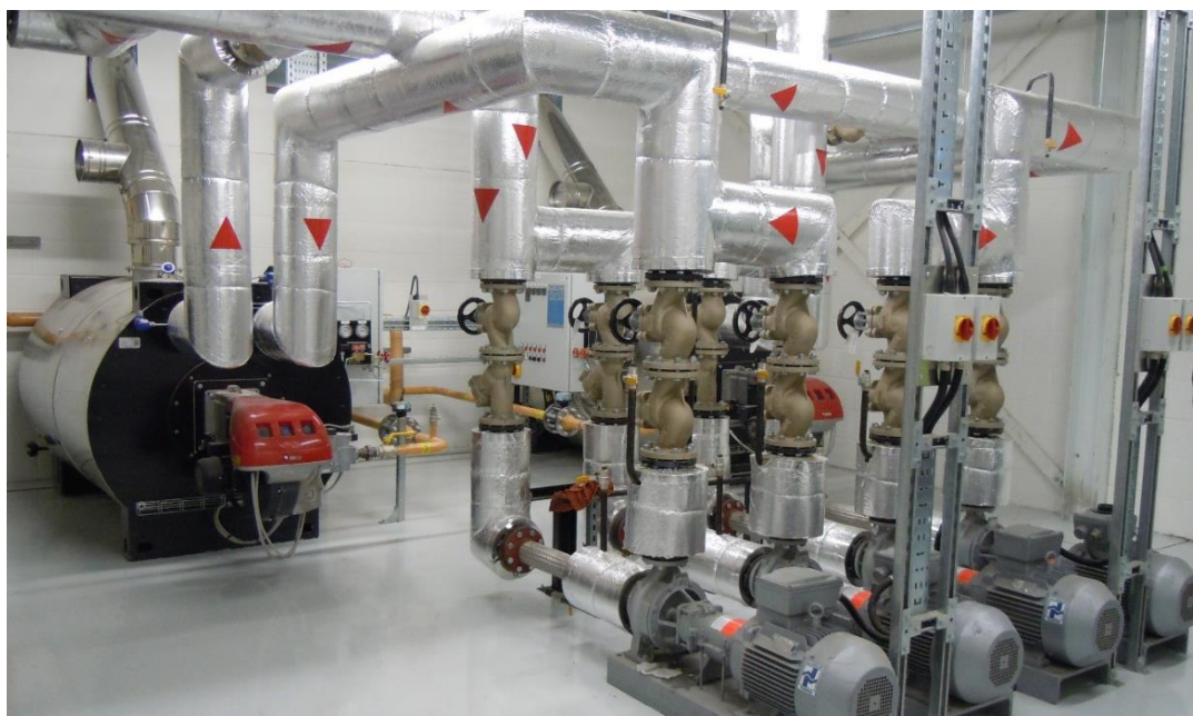
Typical multi-pump thermal fluid installation (Babcock Wanson)
