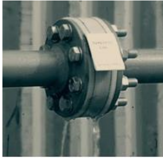
Flange banding installation
