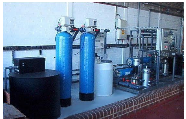
Figure 17 - RO & Water Softening installation
